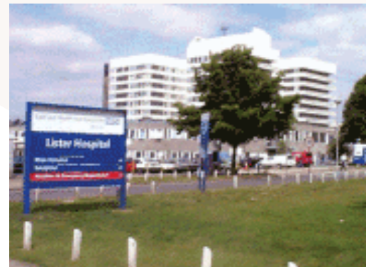
› Lister Hospital, Stevenage, Hertfordshire
