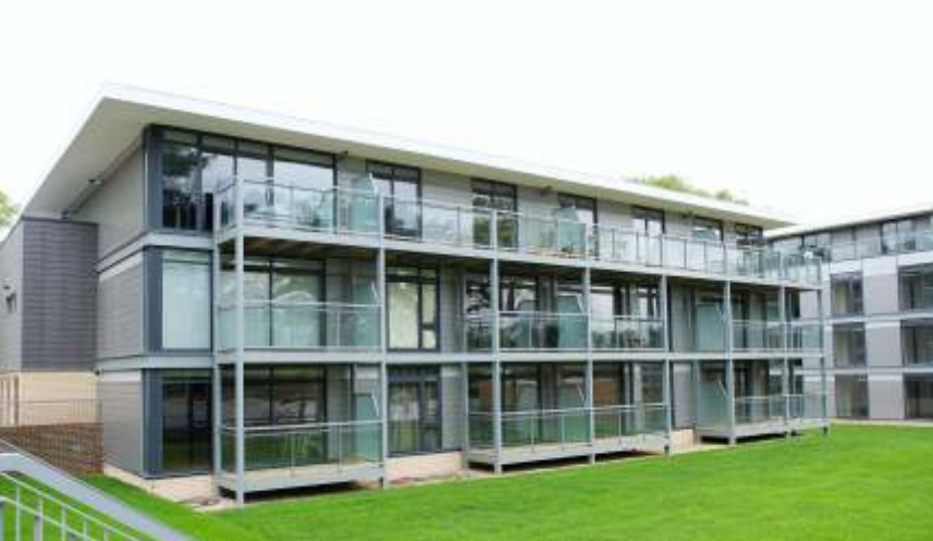
› Former Oaklands College, St Albans (new build)
